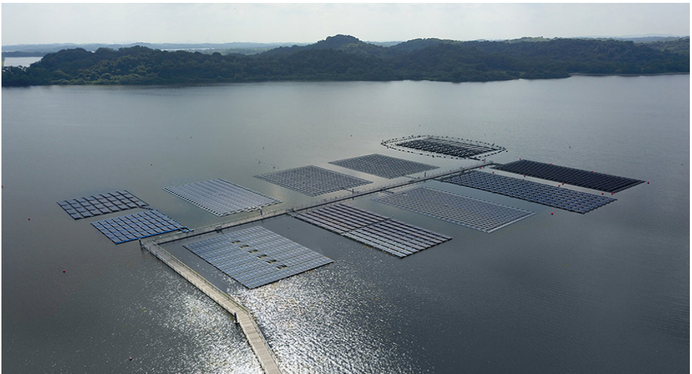
The floating PV system at Tengeh reservoir Singapore comprises different types of floating structures and PV modules of approximately 100 kW p each
