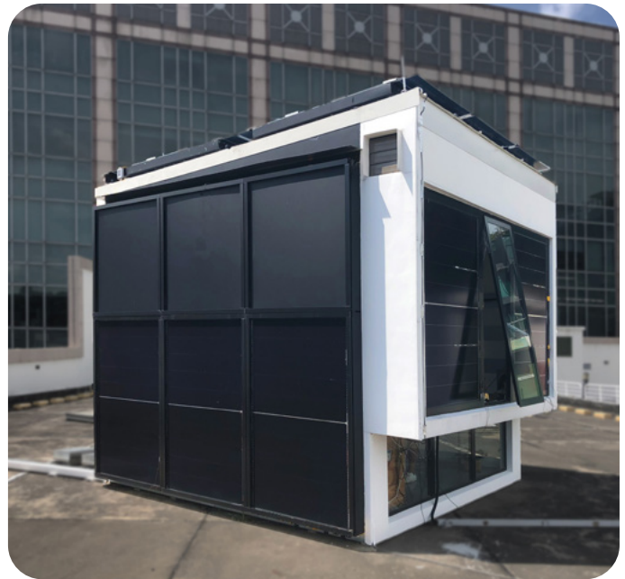
Fig. 1: The patented applied design of a unitised BIPV wall system
