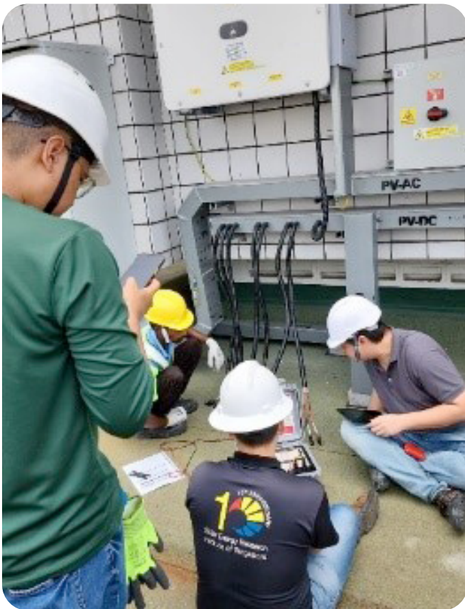
On-site inspection / verification of PV system installations
