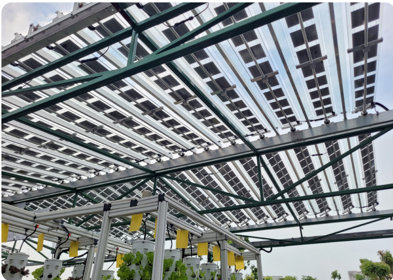
The SERIS Agrivoltaics testbeds have a unique type of PV module which mimics rotatable louvers to track the sun during the day to maximise solar energy generation.
