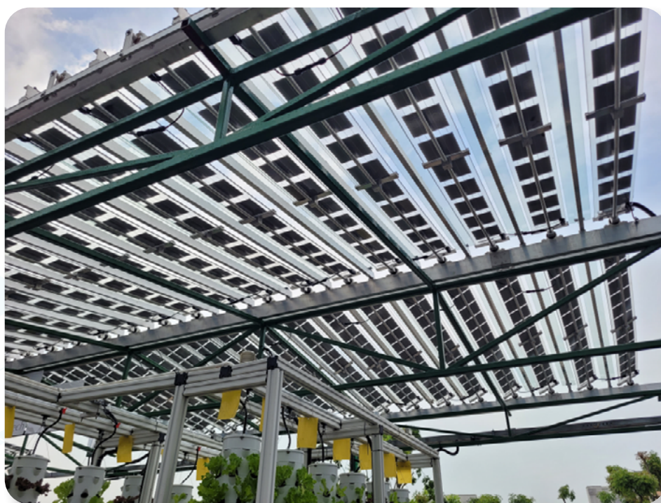
The SERIS Agrivoltaics testbeds have a unique type of PV module which mimics rotatable louvers to track the Sun during the day to maximise solar energy generation.
