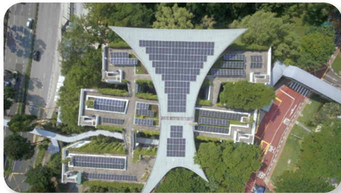
Fig. 1: 135.3 kW p PV system at NUS Ventus. (Image credit: ENGIE South East Asia)
