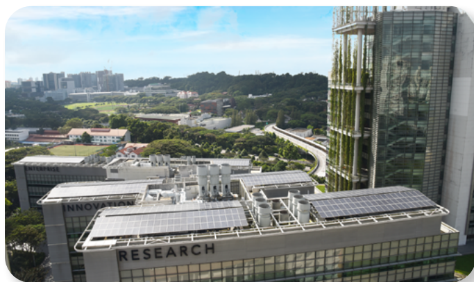
Fig. 1: Photovoltaic systems installed on the rooftops of the CREATE buildings at the National University of Singapore's U-Town campus.
