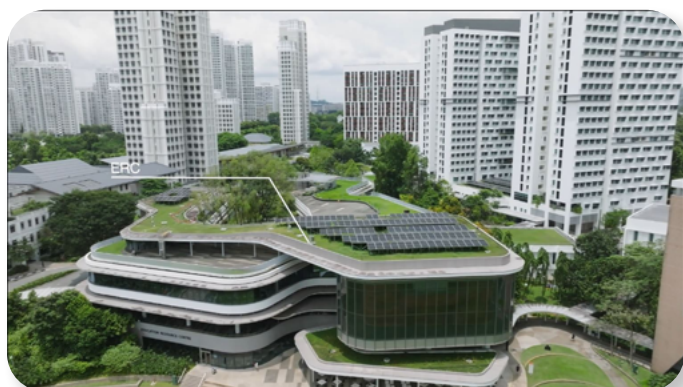
Fig. 3: 128 kW p system at the NUS Education Resource Centre. (Image credit: ENGIE South East Asia)
