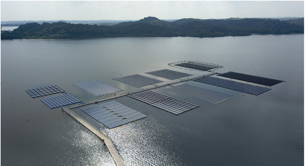
The floating PV system at Tengah reservoir Singapore comprises different types of floating structures and PV modules of approximately 100 kW p each
