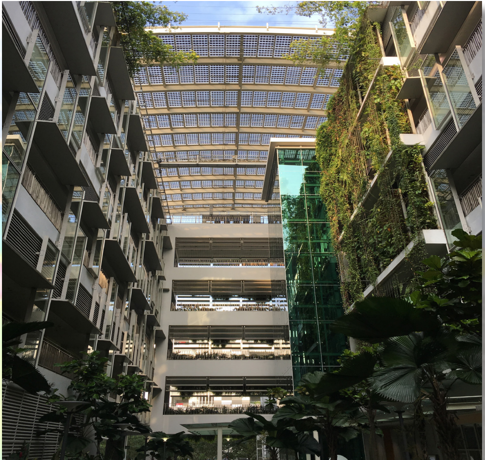
Example of BIPV glass canopy (42 kWp) at Clean Tech One, Singapore: SERIS was technical consultant for BIPV design, tender, component selection and implementation
