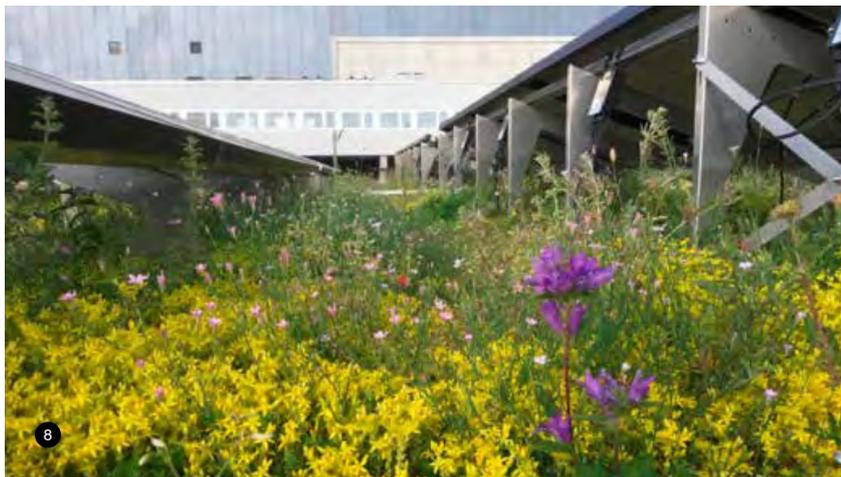
*Figure 5.7: Example of co-location of PV installation with extensive green roof. Source: “Biosolar Roofs” project.*
