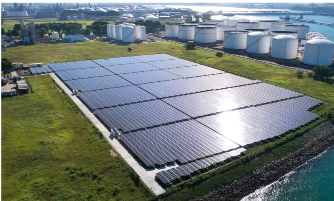
*Figure 5.2: Aerial view of the 5 MWp system deployed by Terrenus Energy on Jurong Island under JTC’s SolarLand programme*
