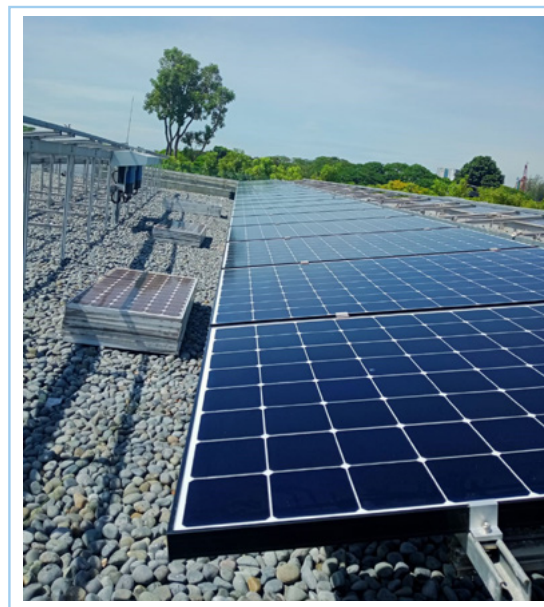
Joint upgrading works by the SST and PVQA groups at the TruePower™ site at Marina Barrage, Singapore. The old solar modules will be tested and assessed in SERIS’ PVM laboratories for their degradation mechanisms.
