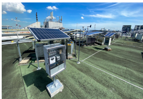
Stand-alone analytical monitoring solution for small rooftops and residential PV systems
