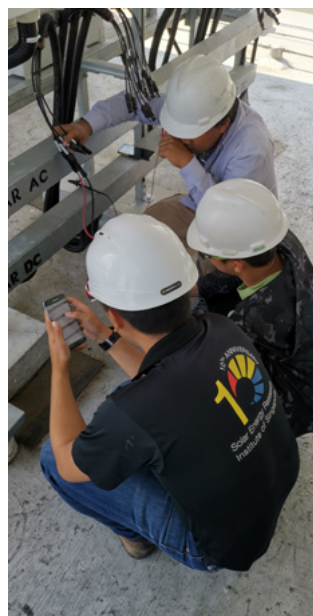
(Left): SERIS engineer performing on-site measurements during testing & commissioning; (Right): Rooftop PV installation on a residential block in Singapore, for which SERIS has acted as Owner's Engineer under the SolarNova programme
