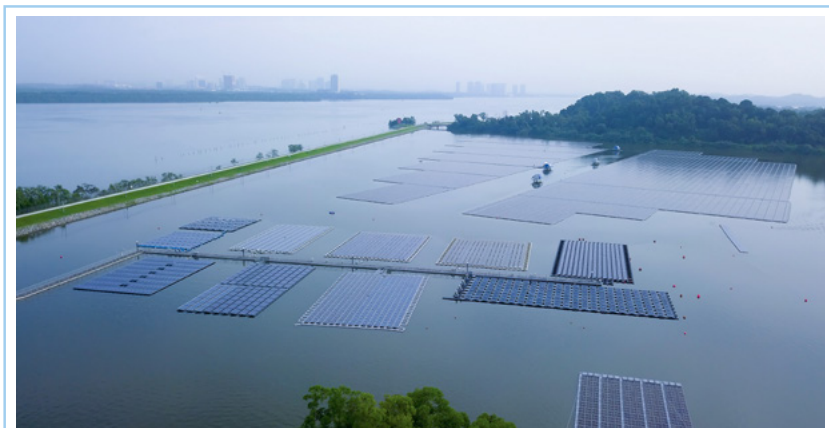
Photograph of Singapore's Tengeh reservoir showing the 1-MWp floating solar testbed (front part) designed and built by SERIS in close collaboration with PUB and EDB. SERIS' scientific evaluations of the 1-MWp testbed were vital for the large-scale deployment of Floating PV in Singapore, including a 60-MWp floating solar farm in Tengeh reservoir built by Sembcorp Solar (one segment can be seen in the back). (Image credit: Sembcorp Industries).
